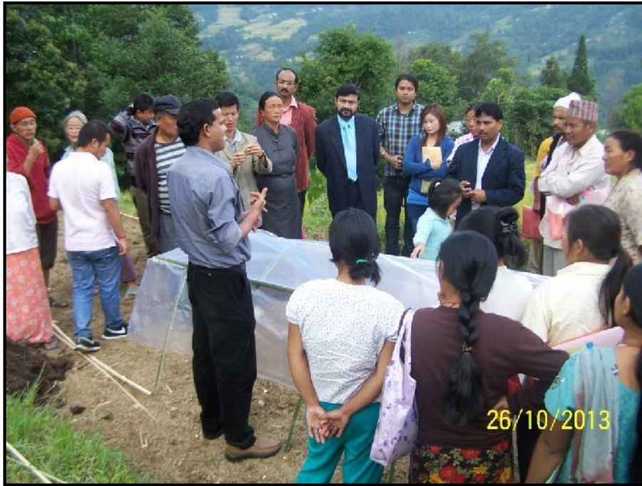
Demonstration of Low Cost Plastic Tunnels Construction to the Farmers
